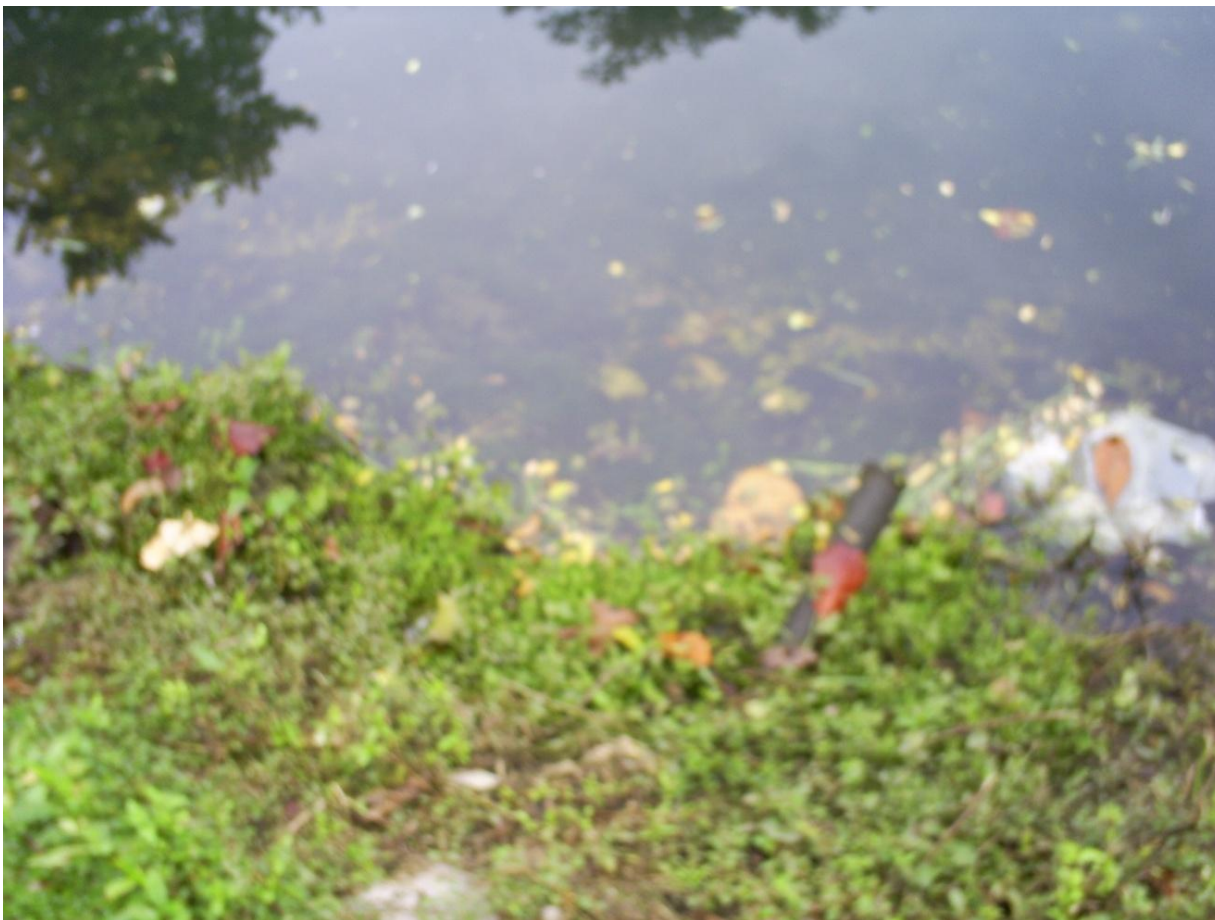
Figure 30. PIC 3 consisted of an unknown pipe sticking out of the ground.
