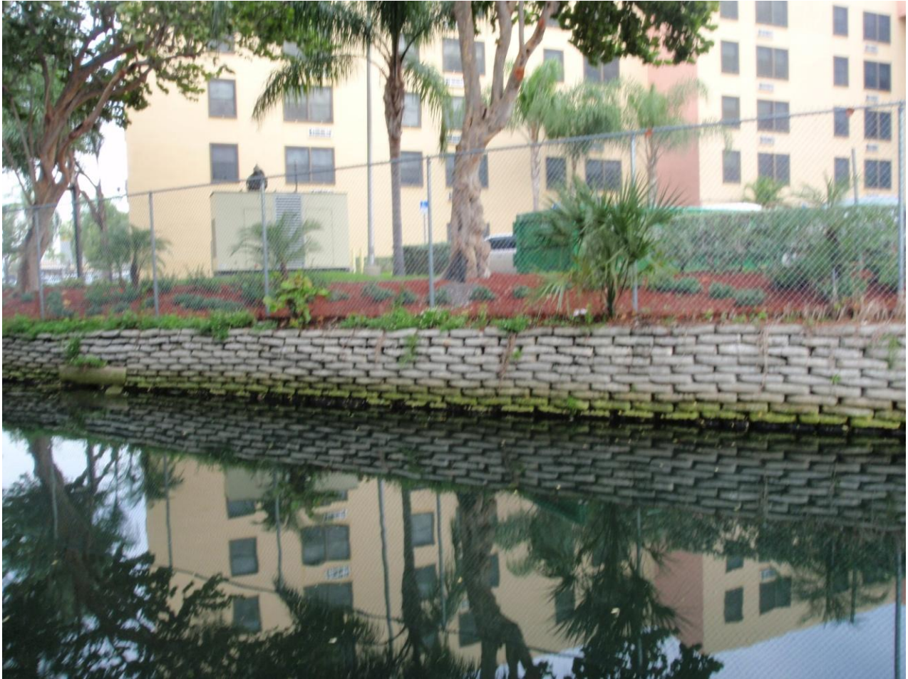
Figure 28. Apartments along the creek at 1310 NW 16 th Street, with private storm drain outlets that discharge directly to the creek; this is a gated community, with no access for an inspection.
