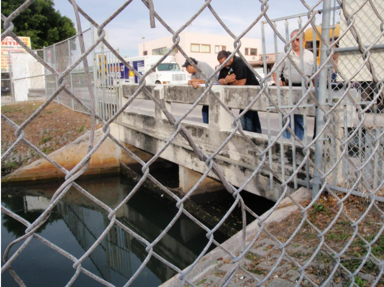
Figure 13. 20 th Street Bridge, where Wagner Creek re-emerges from the underground conveyance.
