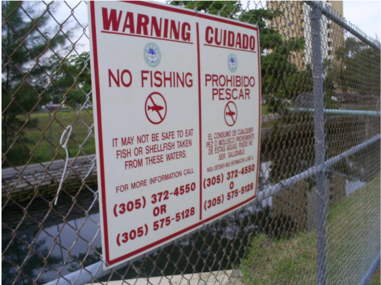
Figure 41. Access to Wagner Creek after the NW 14 th Avenue Bridge is limited, and the team was not able to carry out its inspection because a boat is needed to inspect this area.
