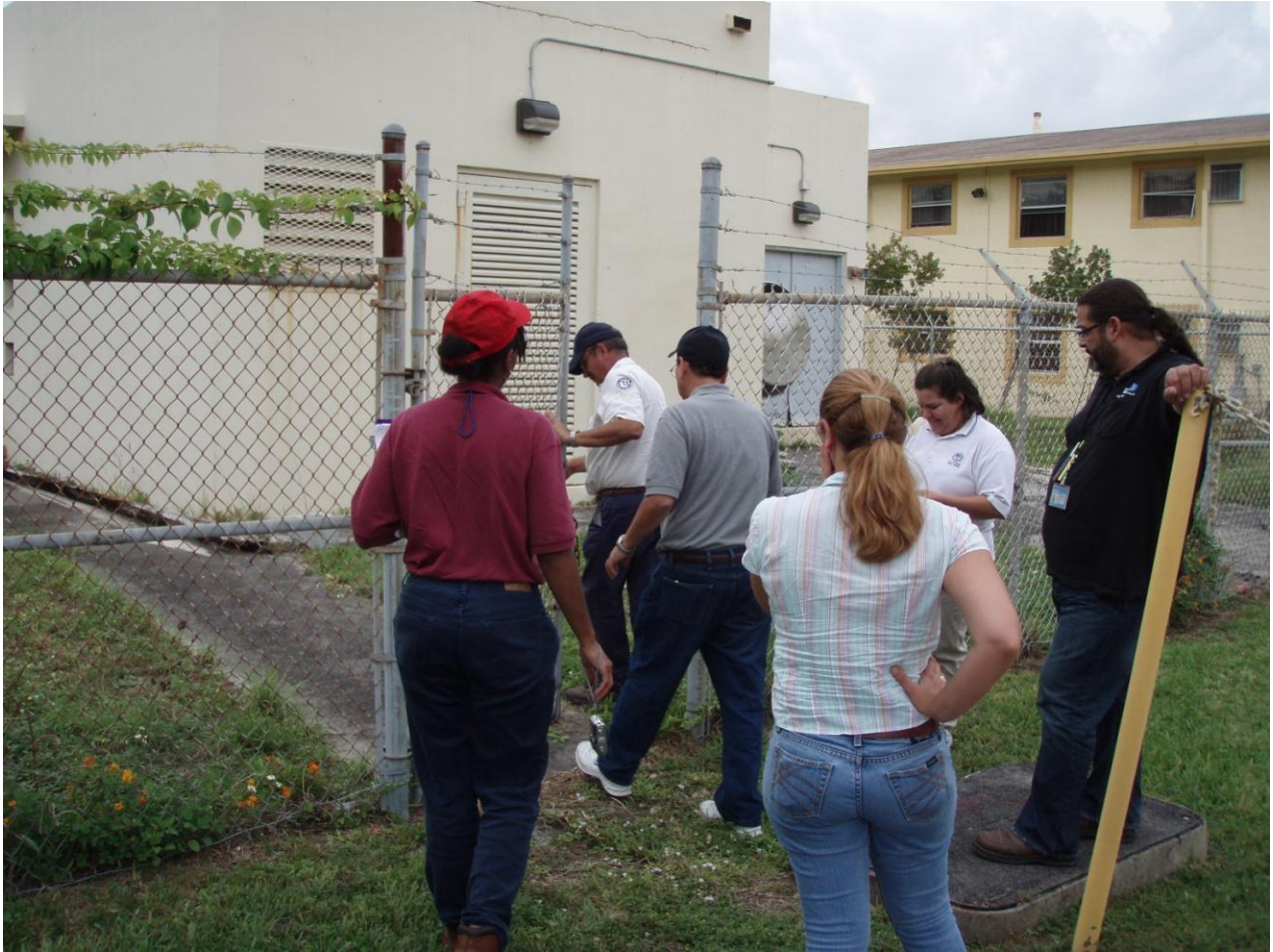
Figure 45. Team members inspecting the City of Miami Overtown stormwater pump station, where construction upgrades are incomplete.
