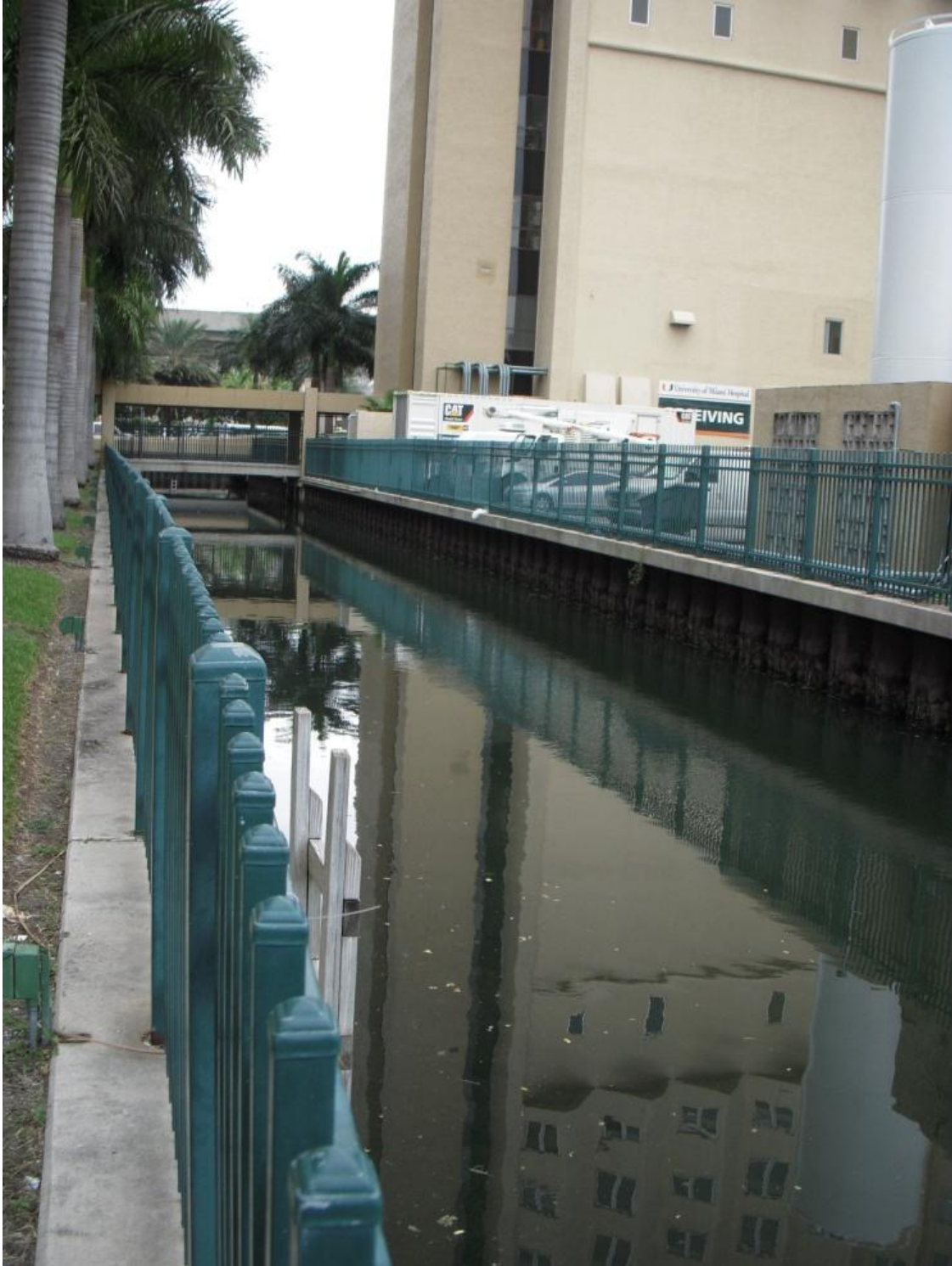
Figure 38. Wagner Creek is channelized next to the University of Miami Medical Center. When the hospital was built, the creek was rerouted to make a 90-degree turn so that there would be enough space on the existing lot to place the hospital building.
