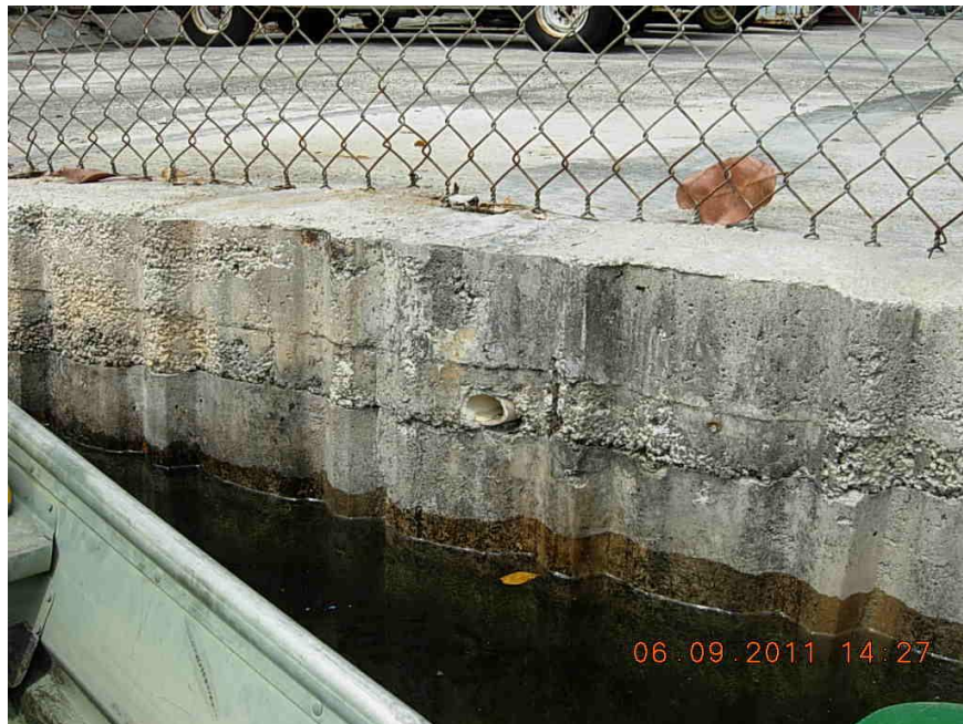
Figure 76. A 1.5-inch PVC pipe originating from Florida Precision at 800 NW 7 th Avenue. GPS coordinates are 25 46' 52.232" N, 80 12' 25.917" W.
