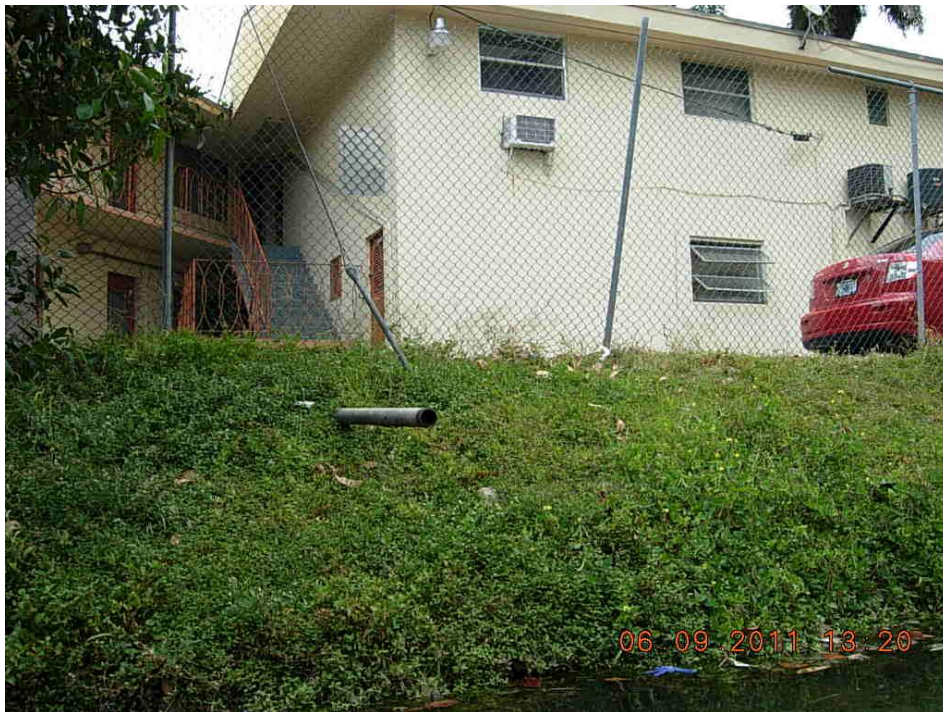
Figure 64. Farther south, two 2-inch diameter metal pipes extended from the same apartment complex. The pipes were within 10 feet of each other. GPS coordinates are 25 47' 36.699" N, 80 13' 15.300" W.
