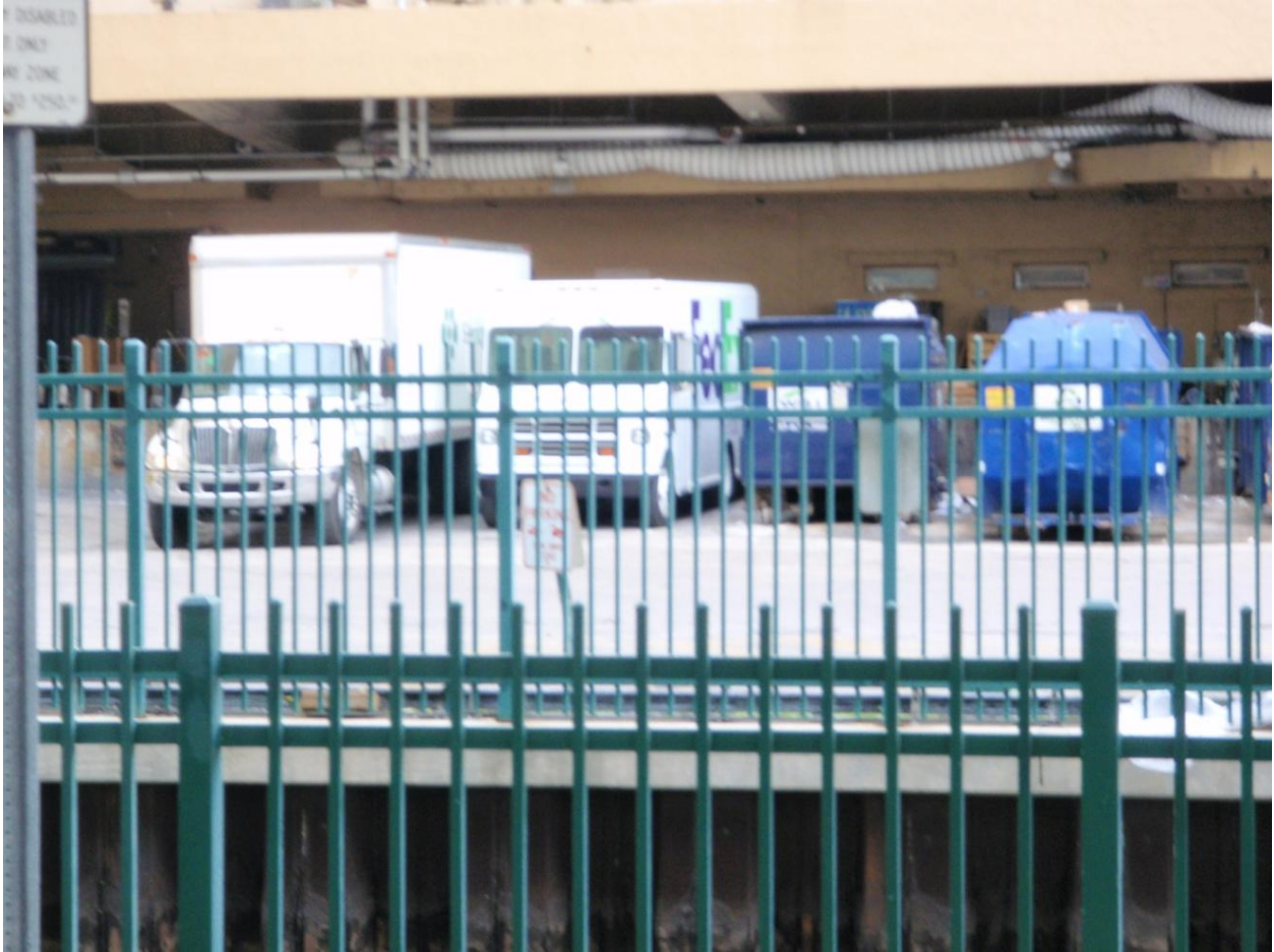
Figure 35. A channelized Wagner Creek flowing past the University of Miami Medical Center, showing dumpsters and trucks right next to the creek, with no berm to prevent untreated stormwater runoff from entering the water.
