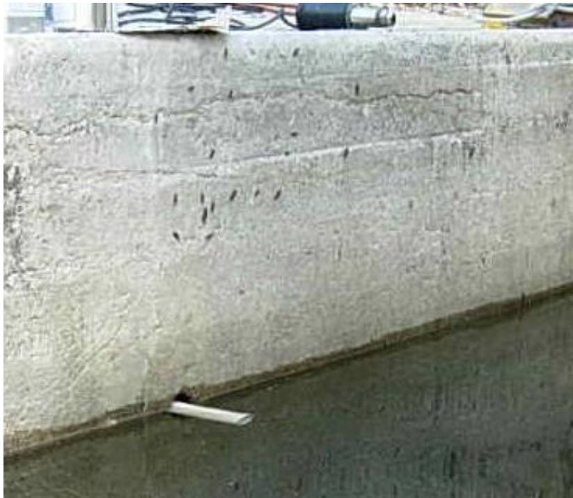
Figure 78. A 2-inch diameter PVC pipe protruding from a private residence. The approximate address is 922 or 938 NW 8 th Street. GPS coordinates are 25 46' 57.121" N, 80 12' 29.900" W.
